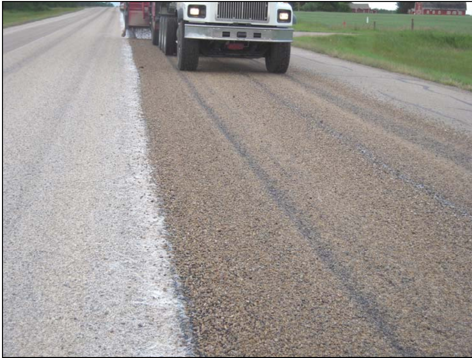
Photo 7. Fibre-Reinforced Membrane with 1 st Layer of Racked-In Aggregate
