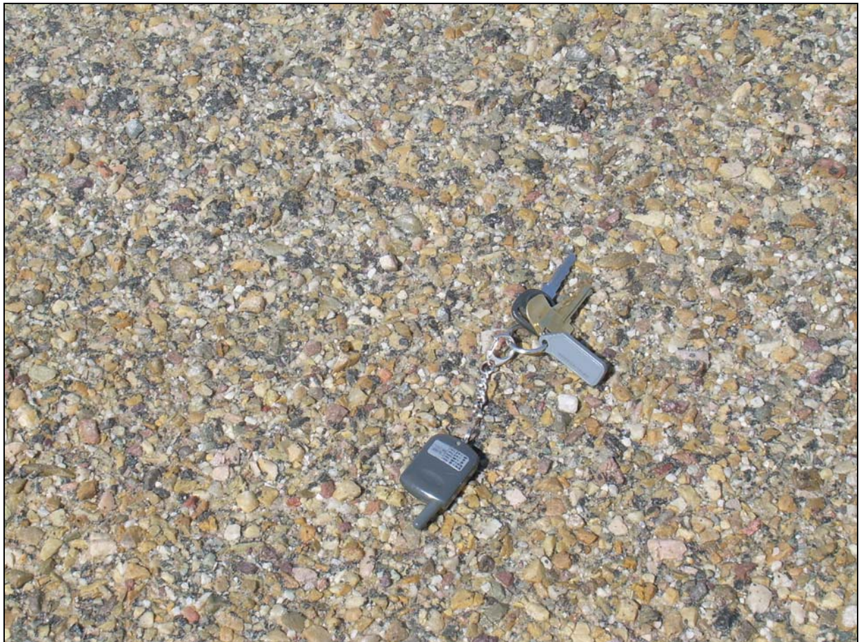
Photo 9. Close Up Appearance of Racked-In Seal (With Fibres)
