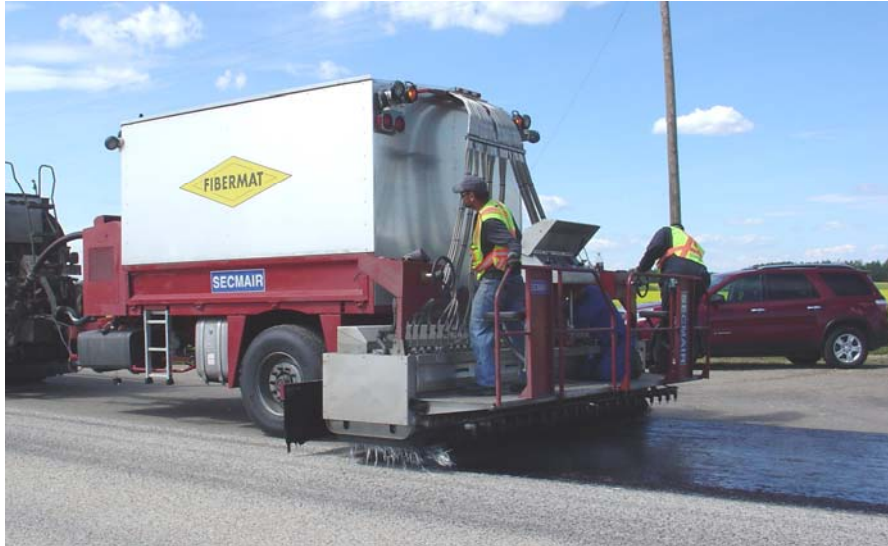
Photo 5. Fibre-Reinforced Membrane Placement Trailer Unit
