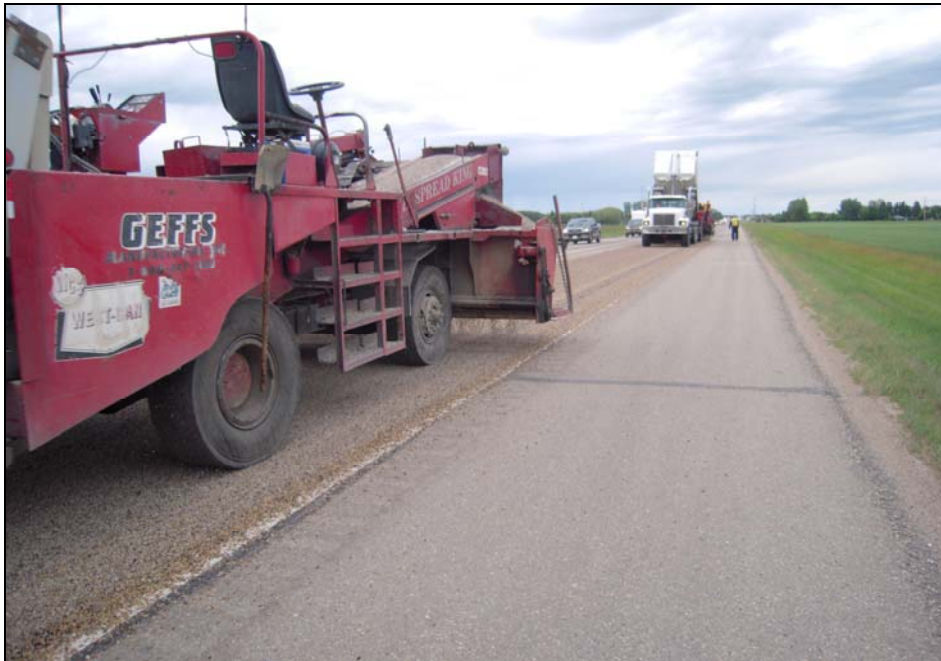
Photo 8. Application of Smaller Chips
