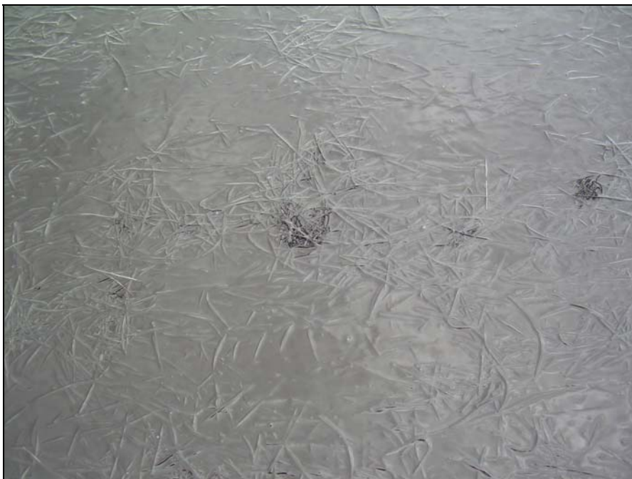
Photo 6. Fibre-Reinforced Membrane Prior to Chip Application
